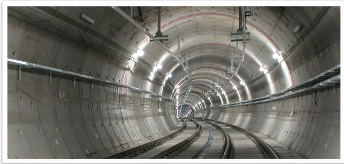
Diagram 7.10 Overhead Contact Rail example (in tunnel)
